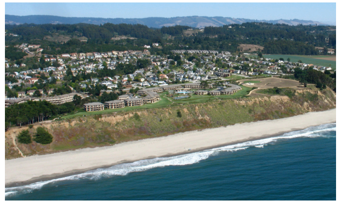
Figure 3.18. Moderately steep sandy bluffs at Manresa State Beach, Santa Cruz County, fronted by a wide sandy beach.
