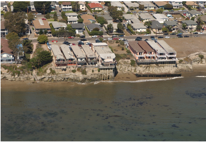
Figure 3.19. Undercut apartment buildings in the Isla Vista area of Santa Barbara County (Kenneth and Gabrielle Adelman, California Coastal Records Project).
