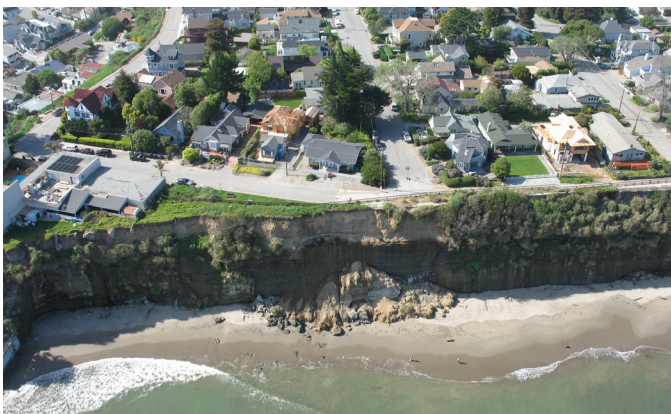
Figure 3.22. Cliff failure on Depot Hill, Capitola.
