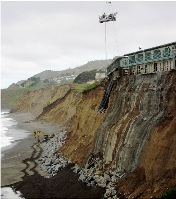
Figure 3.13. Apartments on these cliffs at Pacifica were seriously threatened by wave attack during the winter of 2009-10 and 2010-11 leading to evacuation of the buildings and expensive efforts to try to stabilize the cliffs.
